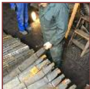
New Boiler Bars in Lancashire Boiler
